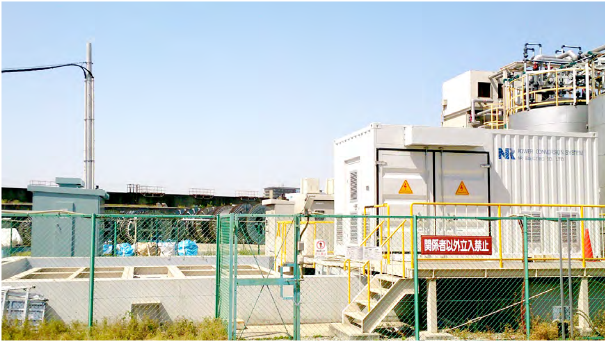
Redox Flow Battery Energy Storage System in Osaka, Japan 1000kW/4MWh Redox Flow BESS
