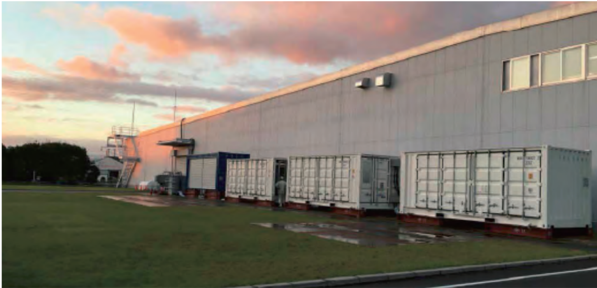
NAS Battery Energy Storage System in Nagoya, Japan 600kW/3.6MWh NAS BESS
