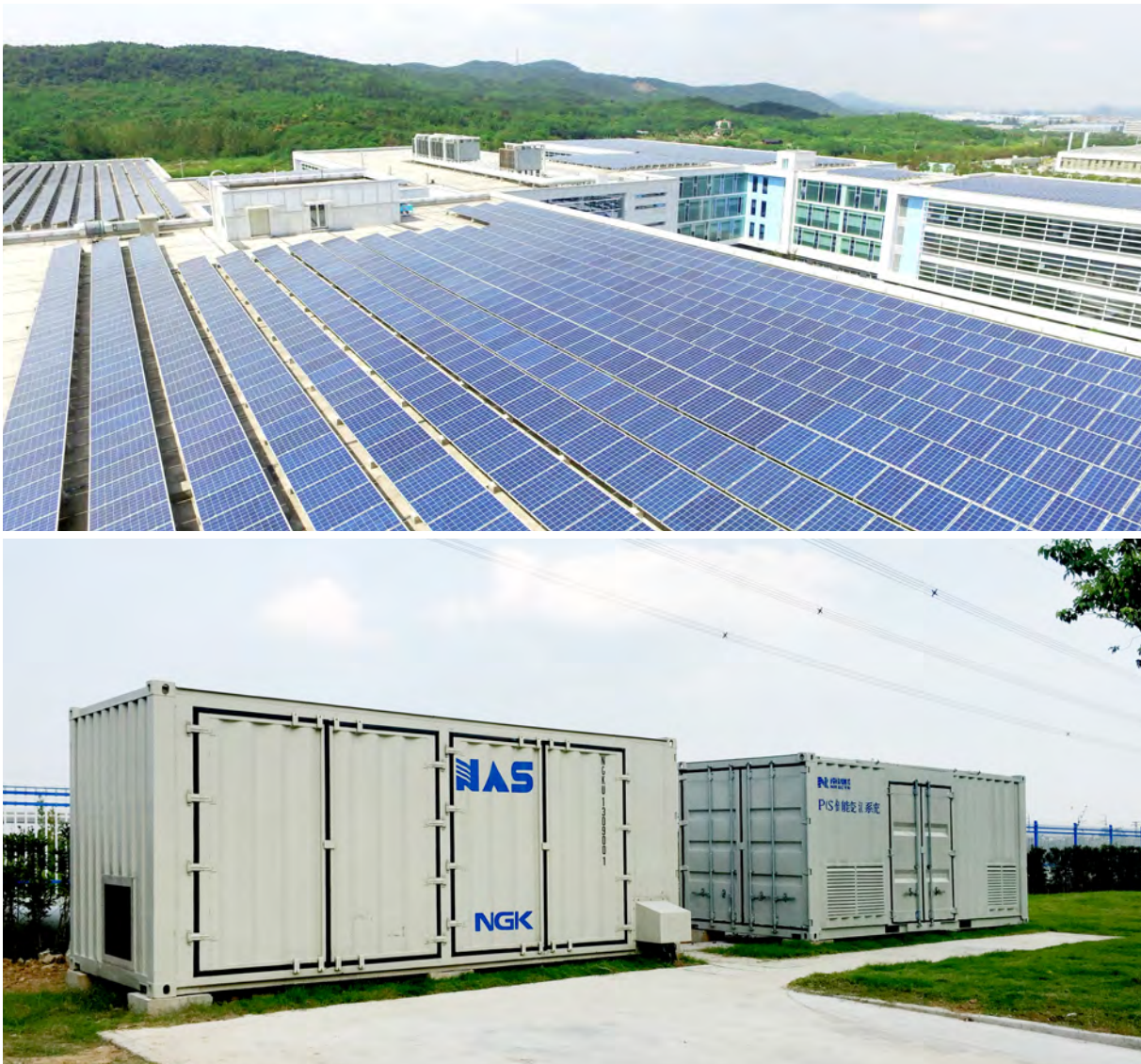
Hybrid microgrid of PV and NAS BESS in Nanjing city, China 2.58MW roof-top PV system and 1.4MWh/200kW NAS BESS
